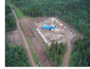
Oil drill on RoadCem stabilization
