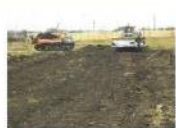
Start of work
