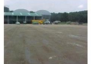
Project overview RoadCem stabilization
