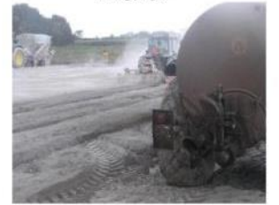
Mixing and spreading of RoadCem
