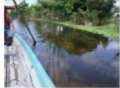
RoadCem construction under water
